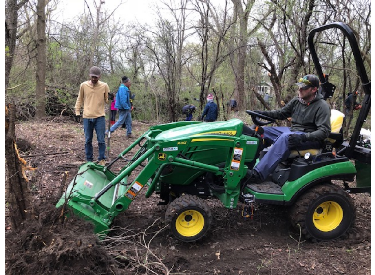
Zupansic Park Clearing by South Hills team
