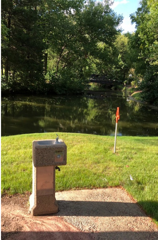
New water fountain and landscape water spigot
