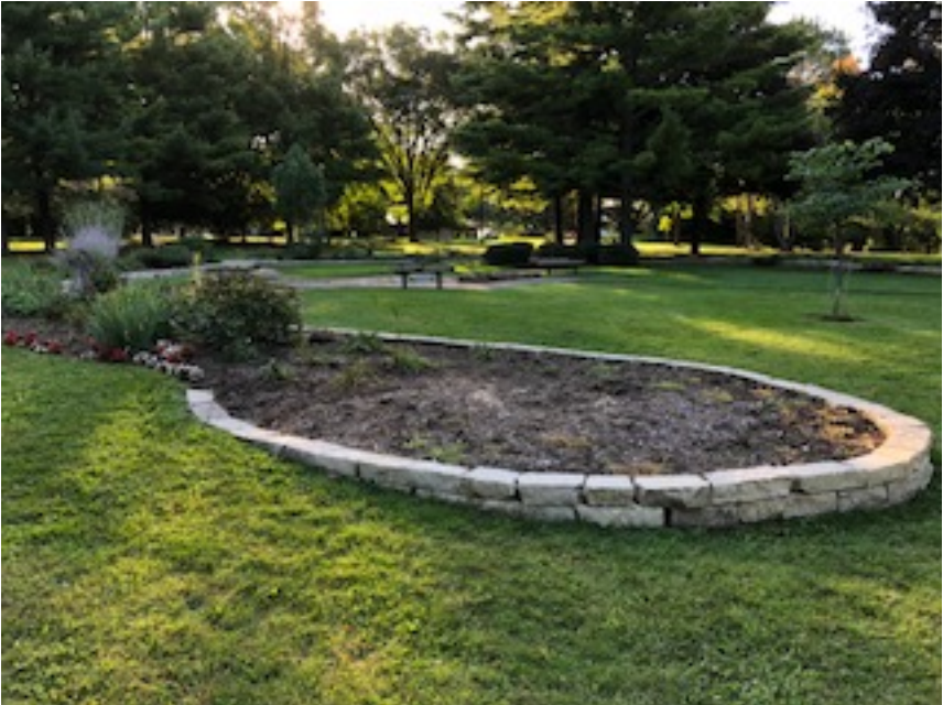
Barsumian Park stone retaining wall restored
