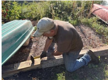
Replaced rotten ties on West side boat launch
