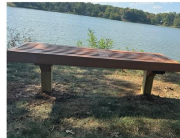
Rest Island bench, and bridge decking repaired
