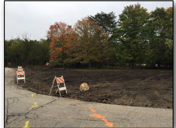
Grading the area at North Lake entrance/Lathan's Landing
