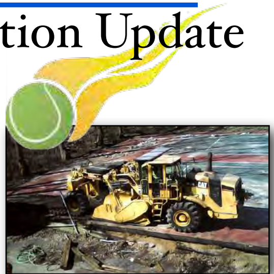
Courts as the grinding of top layers begins
