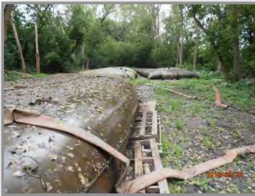
Silt bags located on south shore of Tower Lake
