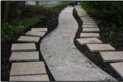
Setting pavers at the east side of the East-West bridge.
