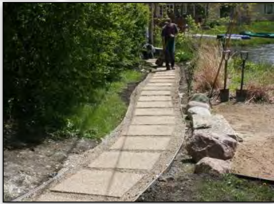
Setting pavers at the east side of the East-West bridge.
